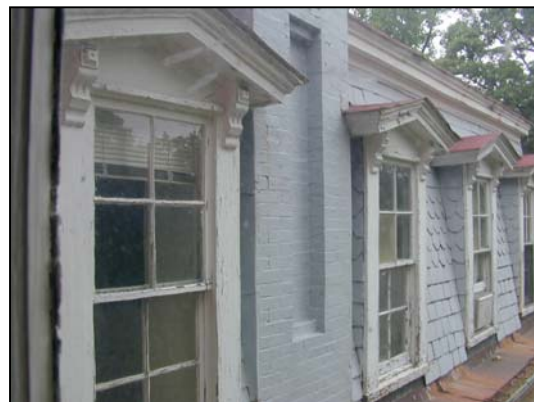
Figure 9 Window detail in mansard roof
