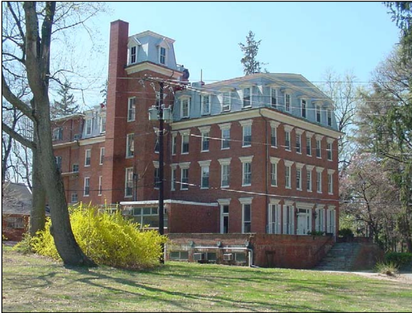
Figure 8 North façade (l) and east façade of Woodlawn Hotel/ Chestnut Lodge building in 2003
